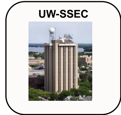
Data Processing Center
