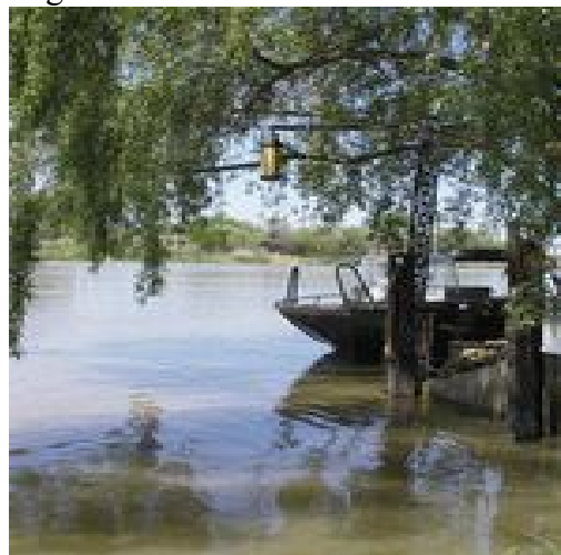
Figure2: Installation of a radar sensor
