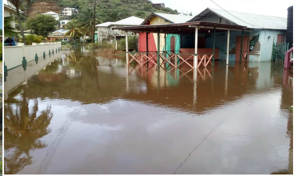
Figure 6: Flooding on Union Island
