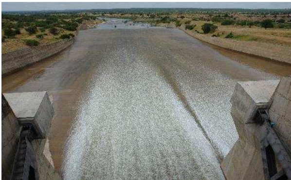
Source: Vogel 2010. Massingir Dam, Mozambique.
