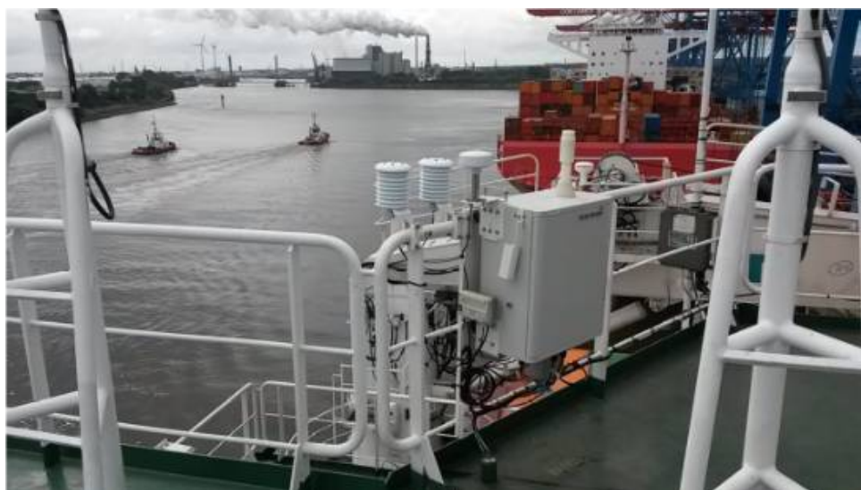
Figure 14: Installation on Montreal Express (DWD)
