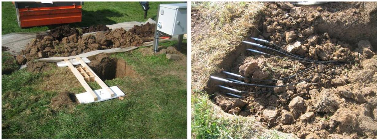
Figure 2. The setup and installation. On the left, the manhole and the template can be seen. On the right, the upper needles and cables are visible above the partially re-filled manhole.
