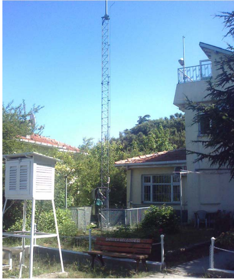
Figure 3: AWOS between buildings
