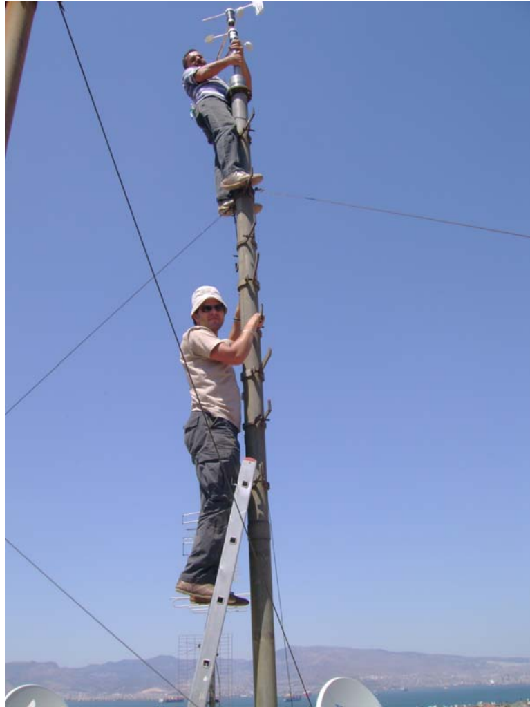
Figure 9: Replacement the oring of wind sensor
