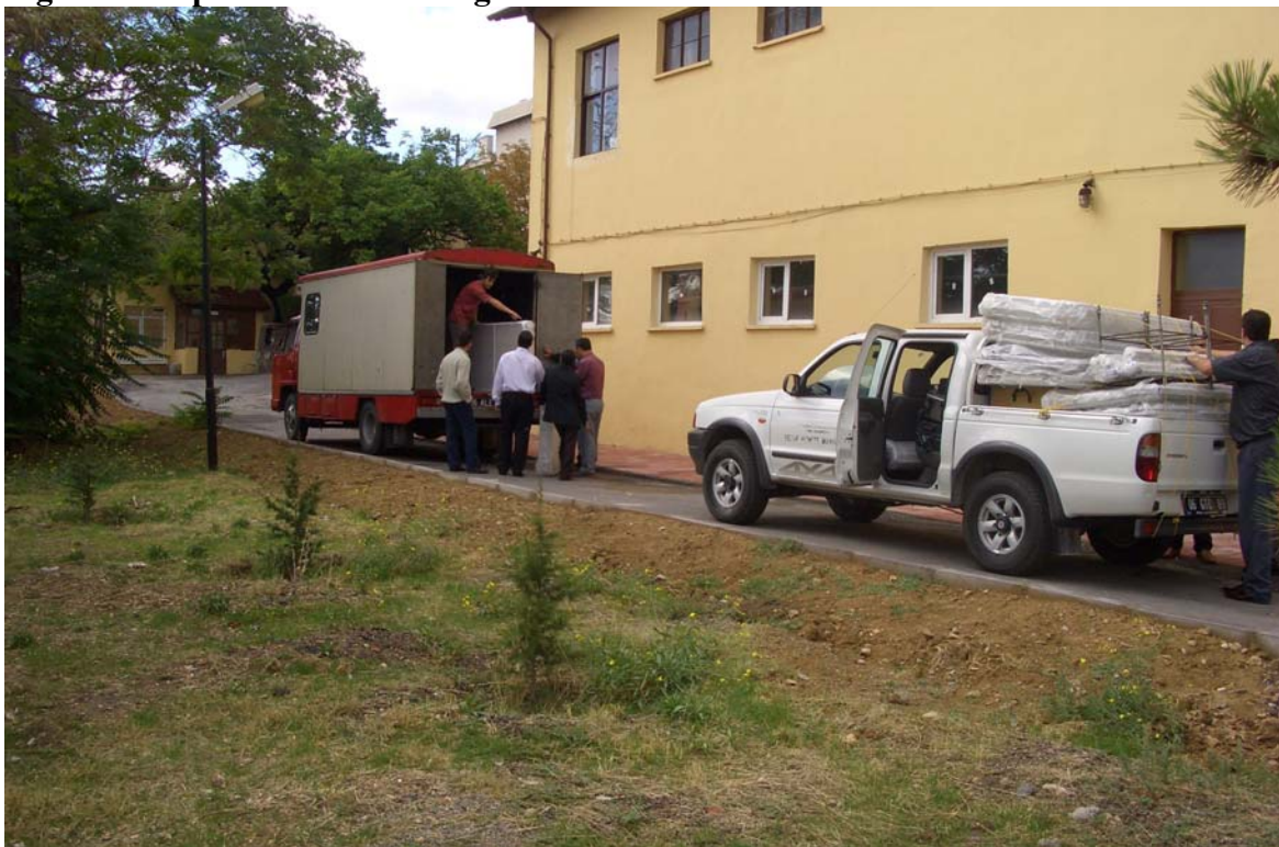
Figure 10: Preparing to journey in order to install an AWOS in a station area
